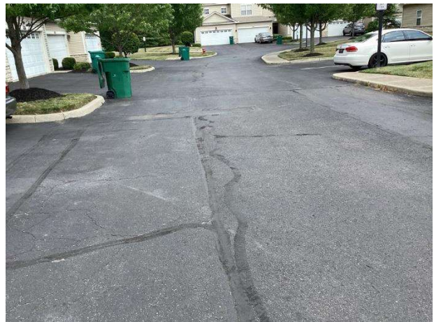
Street pavement overview
