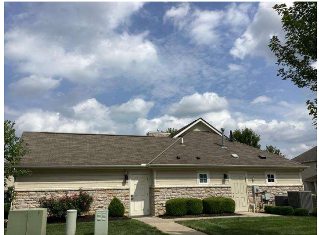
Clubhouse roof overview
