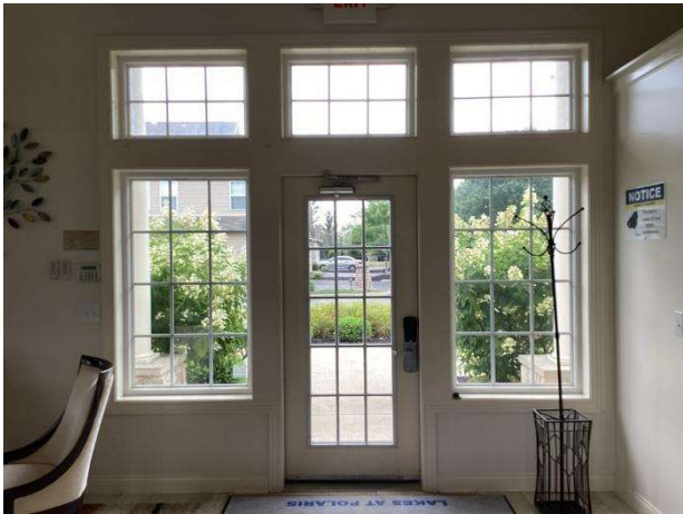
Windows and door overview
