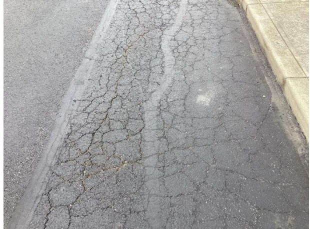
Alligator cracks
