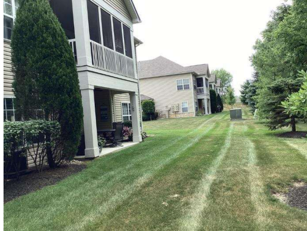
Area to install subsurface drainage behind Buildings 5 and 6
