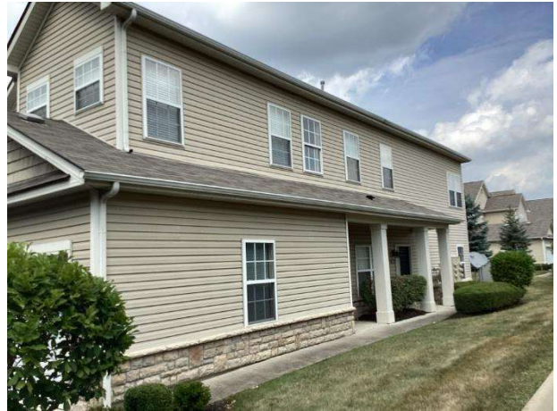
Vinyl siding overview
