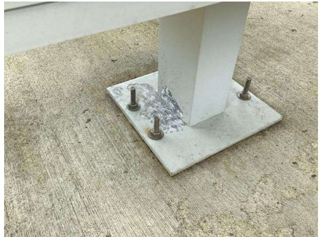
Finish deterioration
