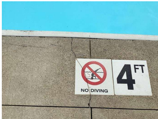
Concrete cracks
