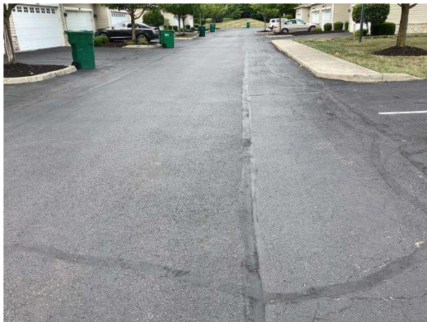
Street pavement overview
