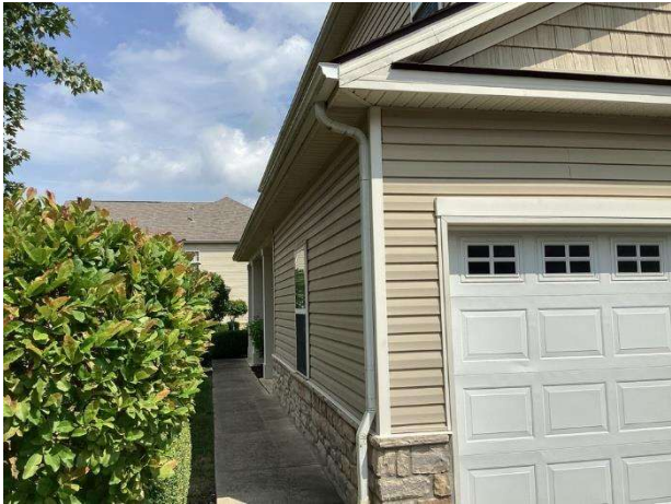
Gutter and downspout overview
