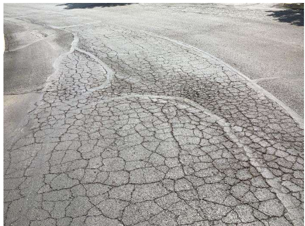
Alligator cracks
