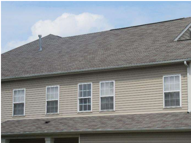
Residential building roof overview
