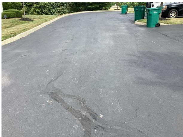
Street pavement overview
