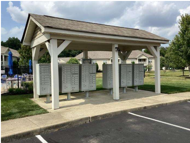
Mailbox stations and enclosure
