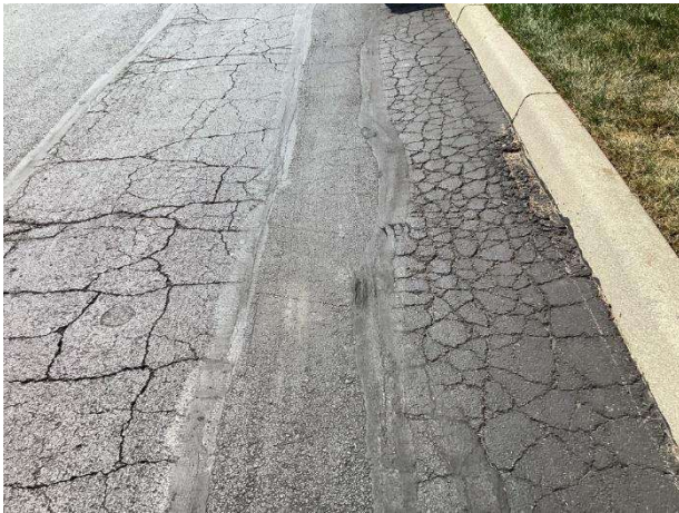
Alligator cracks
