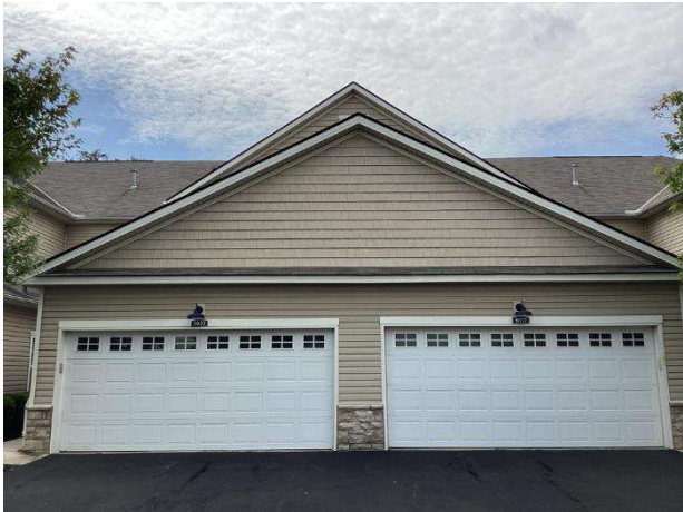
Vinyl siding overview
