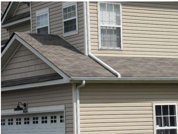
Isolated downspouts routed to lower gutters
