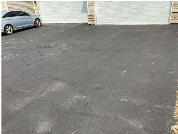
Driveway pavement overview
