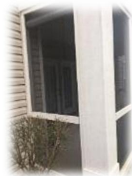
Exterior, Side of Screened Patio
