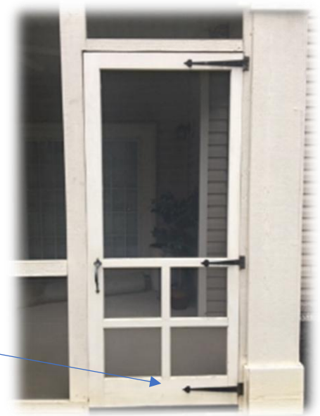
Patio Screen Door Installed
